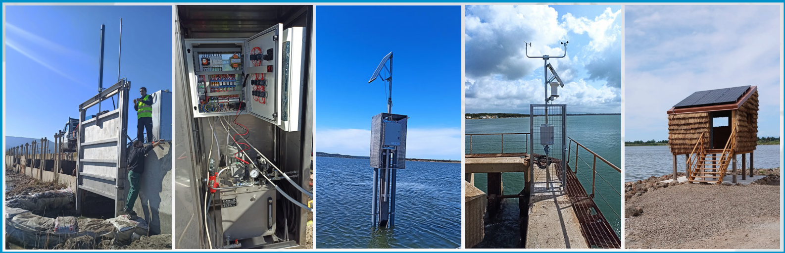
Smart Gate installation
