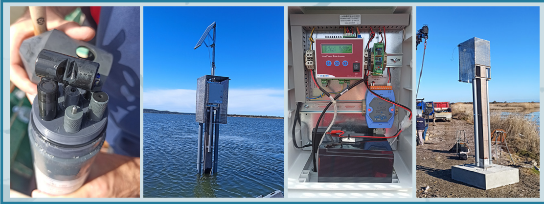
Probe detail View of Station B Data logger Support structure
